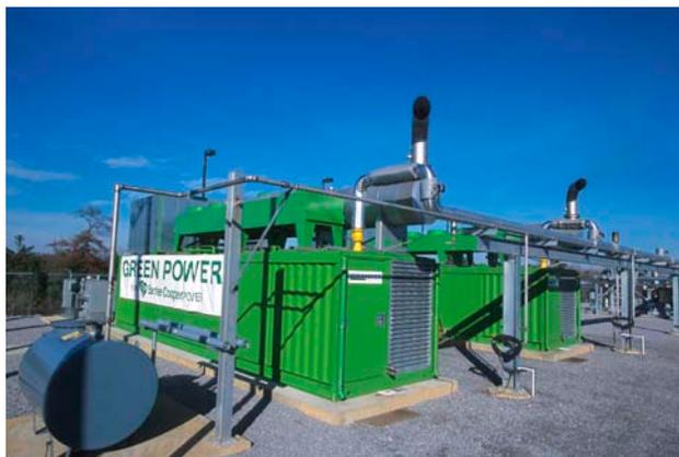
One of the five landfill electricity generation plants around South Carolina built by Santee Cooper. Methane, a potent greenhouse gas, is captured from the landfill and used as fuel to power the generators that produce the electricity. At this time, it is more expensive to install this kind of facility than traditional power plants. However, this could change over time.
