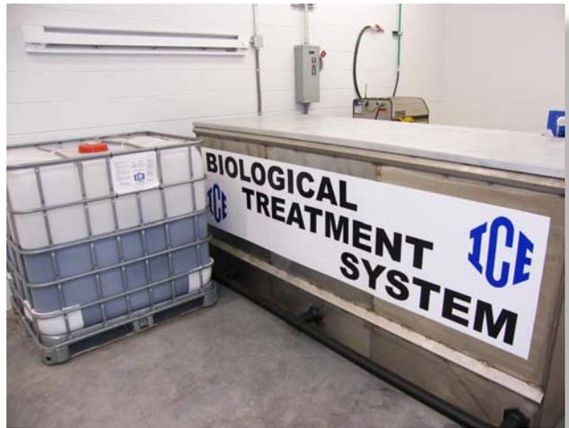
The stainless steel tank is where the bugs live. Millions of microbes clean the water of oil and soap deposits. The tank on the left is where the final filtration of the recycled water takes place. Next stop, another dirty truck.
